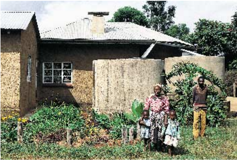
In Kenya, rainwater is harvested from roofs and stored in tanks, a simple technical solution that can help solve water quality and quantity problems, and reduce time needed to fetch water.
