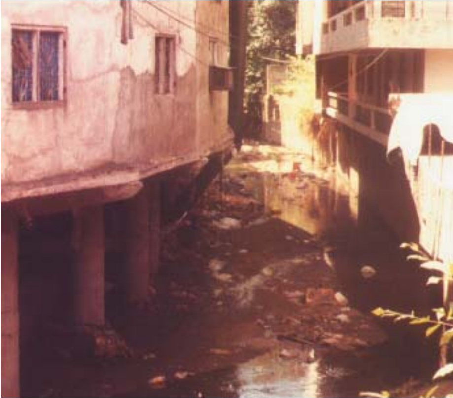
Construction of houses from both banks almost obliterates Pinga Oya, and river constriction causes major flood damage.
