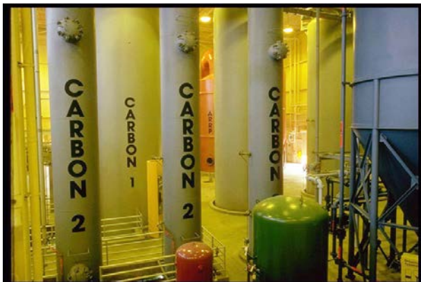
Two-stage granular activated carbon adsorption contactors at Denver Potable Reuse Demonstration Plant
